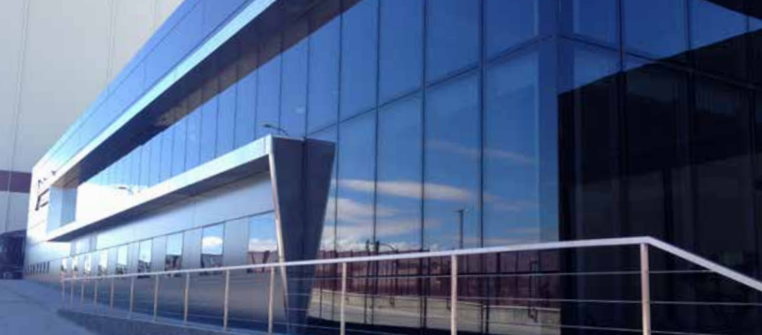
Qbiss Air, Glass Curtain Wall System
